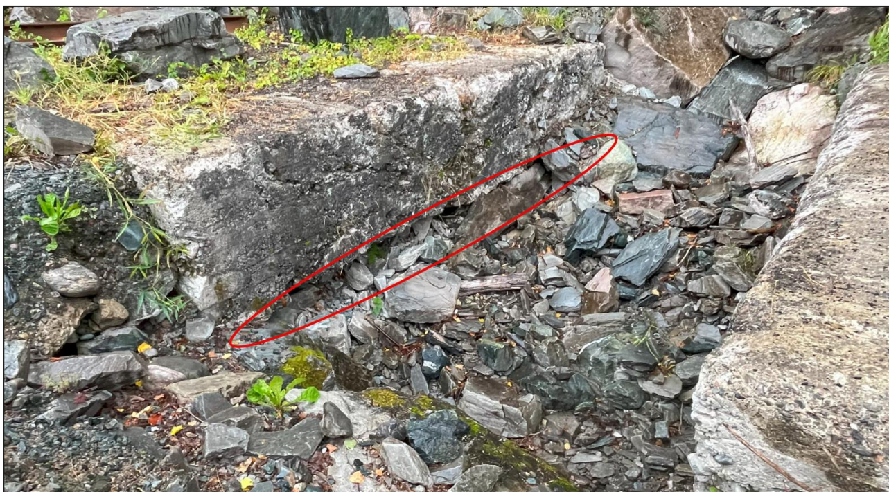
Figur 7. Undergravd betongkulvert.
