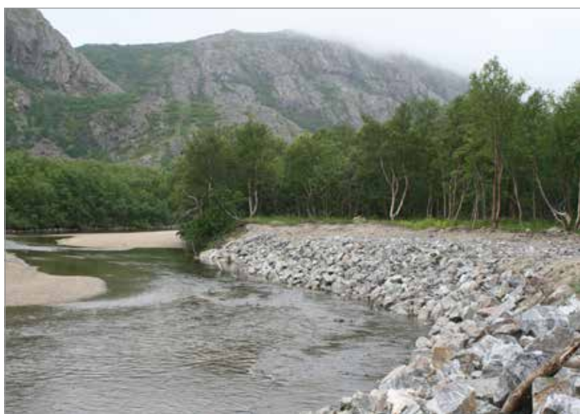
Erosion control structures in Grense Jakobselv River. Photo by Natalia Polikarpova.
