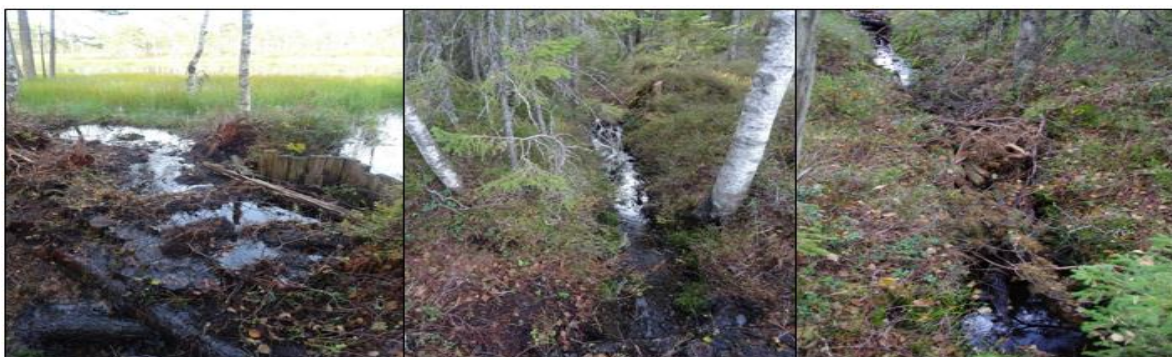
Figure 4. The status of ditches at location C at lake Vatnartjerner in Northern Kisselbergmosen peatland after heavy precipitation in September 2015. Photo: David Arnott
