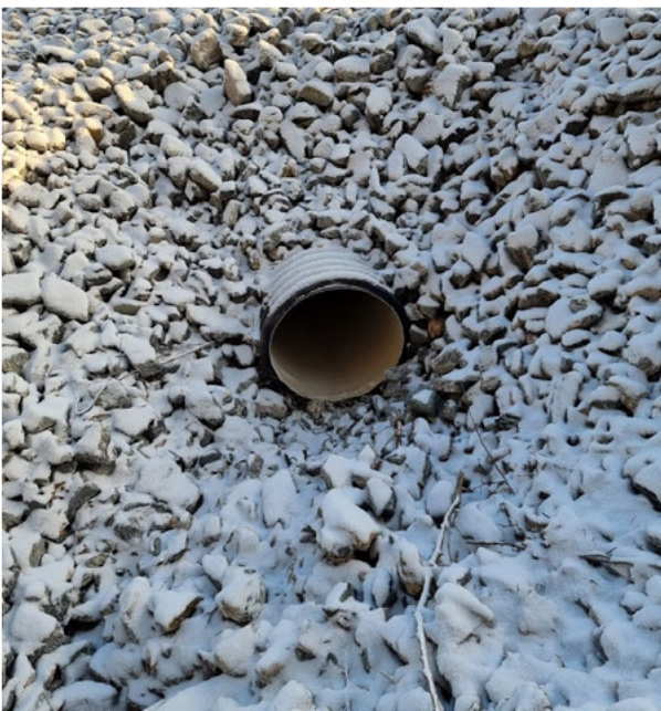
Figure 5 The existing 600 mm smooth HDPE culvert under the landfill.
