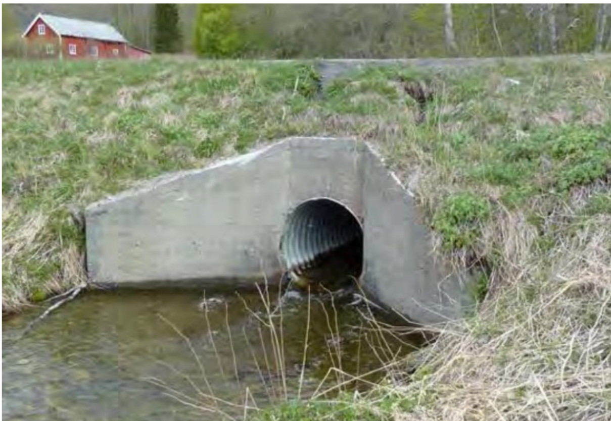
Figure 7 Example of V-shaped culvert intake.
