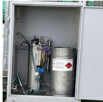
Figur 8 : Lagertanker for Tetrahydrothiophene.
